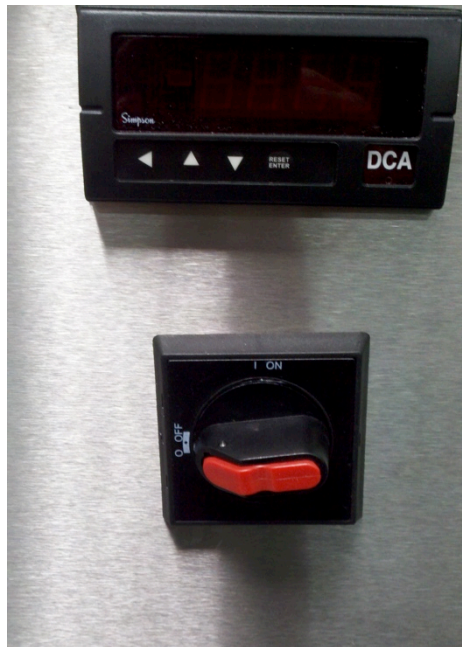
Figure :Showing the position of the Rectifier Disconnect Switch in the OFF position
